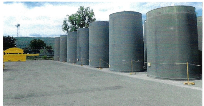
Figure 3 Spent nuclear fuel canisters are stored inside concrete overpacks to block radiation.
